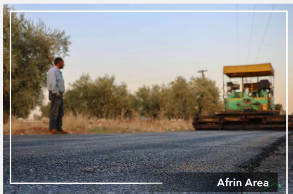
Paving the Road to Afrin National Hospital
